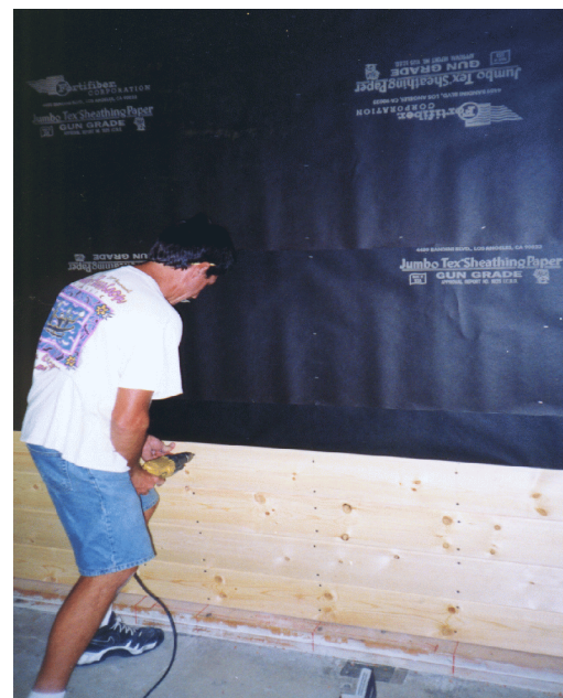
Figure 51 Application of 1" x 8" pine planks to stud wall.
