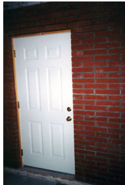
Figure 54 Appearance of brick facade with door installed.
