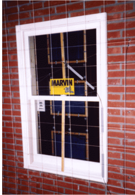
Figure 56 Appearance of brick facade with window installed.
