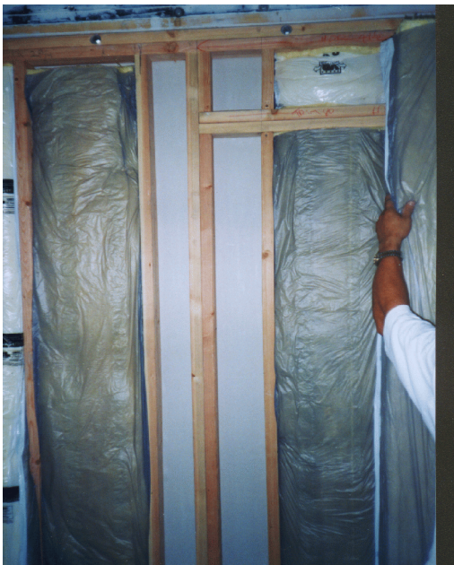
Figure 50 Installation of fiberglass insulation batts between stud wall uprights.
