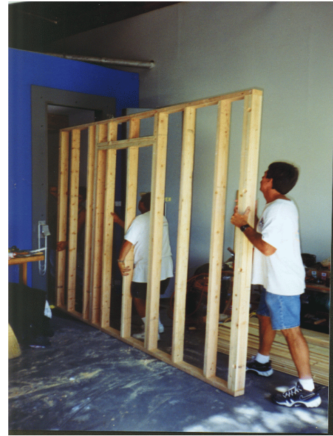
Figure 49 Installation of stud wall frame in low-frequency test facility.
